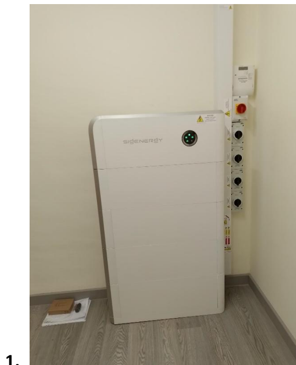
Solar battery storage unit
