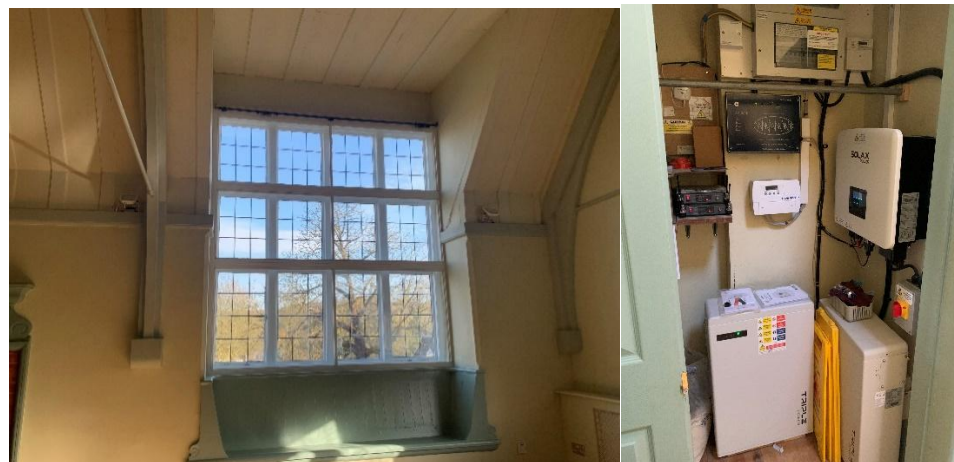
Newly installed secondary glazed windows and battery storage unit for the solar panels
