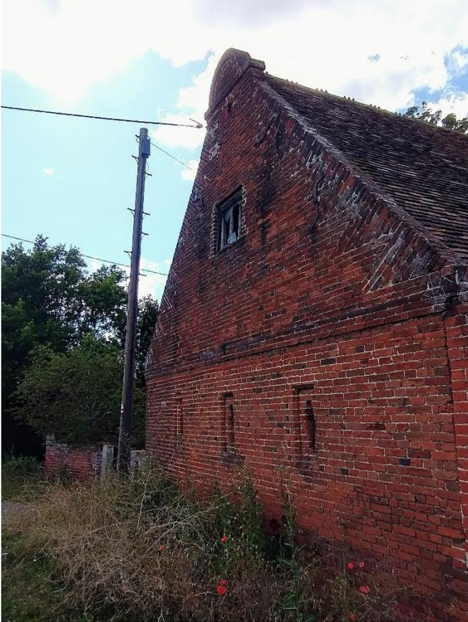
The handmade bricks laid in the expensive Flemish bond, tumbled-in brickwork, the decorative ridge tiles, moulded window surrounds and semi-circular gable apex are all features included to raise the aesthetics of the barn beyond the purely functional.
