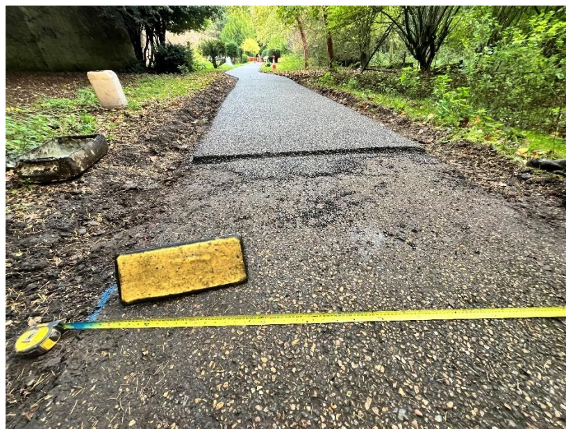
The Flexipave surface under construction
