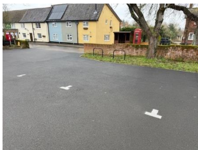
Mendham – Improvement of car park
