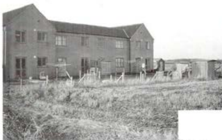
▲ Unscreened rear gardens.
