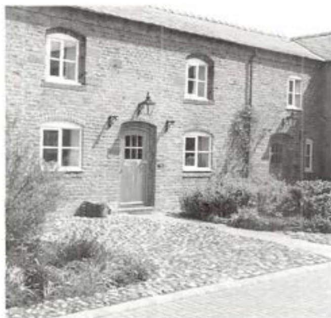
Traditional detailing - simple grid of windows over windows
