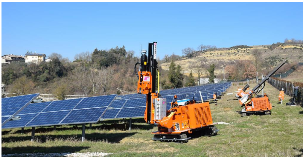
Image 1: Typical GPS Solar Farm Pile Driver
