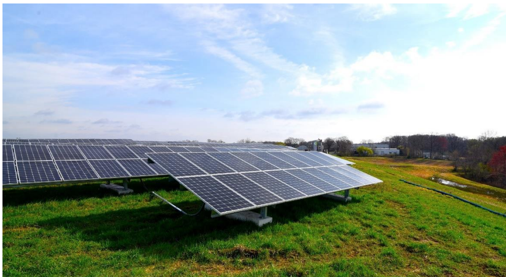
Image 4: Typical ‘No Dig’ Solar Panel Installation
