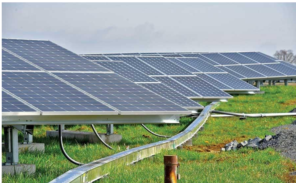
Image 5: Typical 'No Dig' Solar Panel and Cabling Installation
