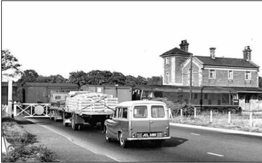
figure 57: C21st Images of the Hadleigh Branch Line crossing the A12
