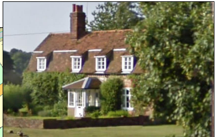
◀ Pond Hall Grade II Cottage. C16 or earlier timber frame with C18 red brick facing. C20 matching bay to left
