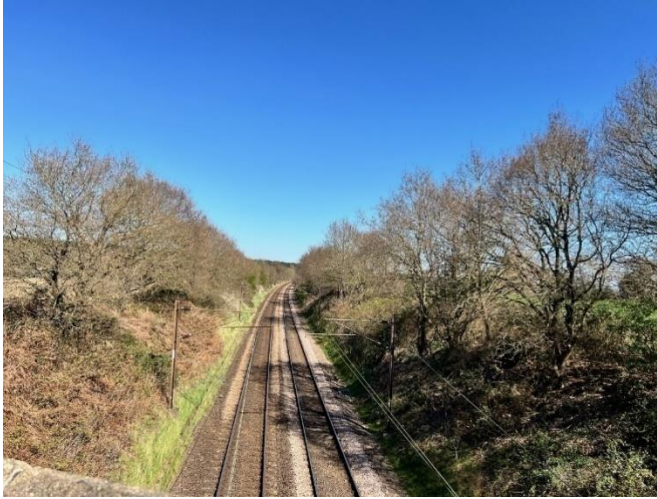
figure 62: Mainline in Cutting from Bridge in the PBCA
