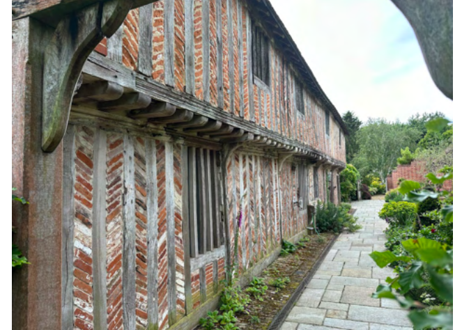
Plate 11 Bentley Hall Stables/Meeting Hall showing herringbone brickwork and closely spaced joists.
