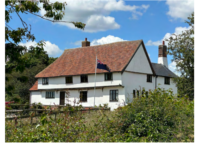
Plate 23 Hubbard's Hall, grade II listed building dating to the 16th century.
