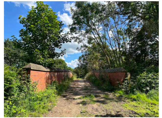
Plate 20 Railway bridge with earlier fabric at track level.
