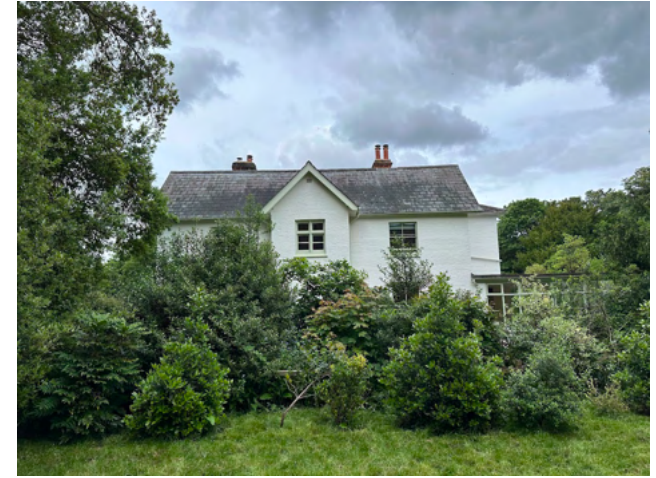
Plate 5 Bentley Church House as seen from the church yard to the south.
