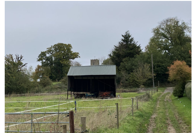
Figure 42: Placement of small agricultural building restricting the view of Baylham Church from a prominent public right of way which is to be discouraged.
