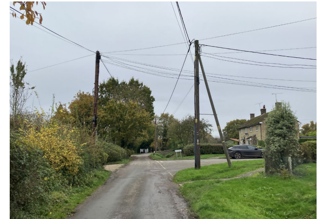
Figure 03: Church Lane. Note general design guidance on page 31 regarding community aspirations for the management of overhead cables.
