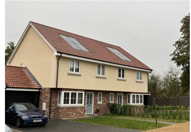
Figure 52: Contemporary property with subtly placed solar panels incorporated into the roof design.
