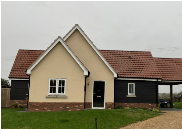
Figure 37: Contemporary house design with use of black weatherboard and light colour render which integrates well with Baylham's vernacular and rural Suffolk setting.
