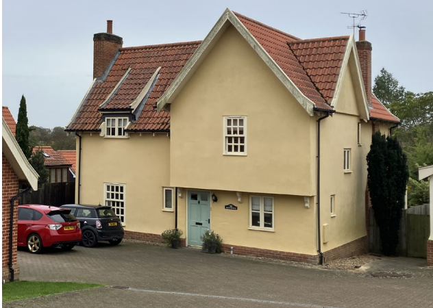
Figure 35: Contemporary home with traditional architectural features including a high roof pitch, deep recesses within the eaves and sash windows with glazing bars.
