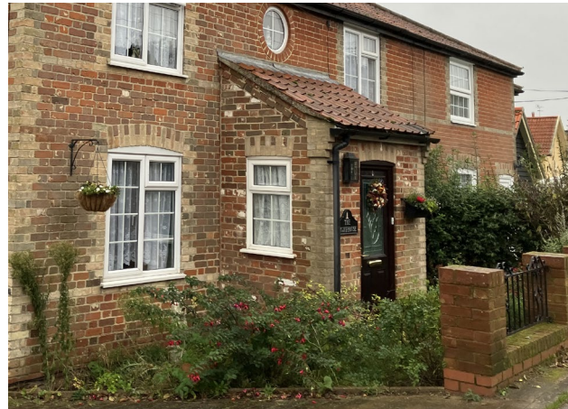
Figure 61: Example of low brick walls and iron fencing, permissible as a quality boundary treatment.
