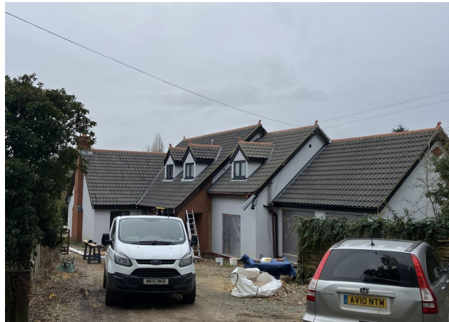
Figure 38: An additional example of a contemporary home under construction with contemporary iterations of traditional features, including colour render, narrow gable dormers and glazed slate pantiles.
