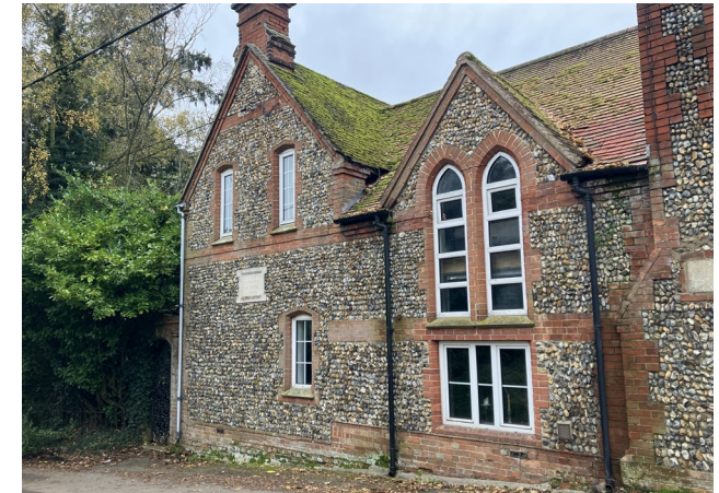
Figure 14: The National School with flint walls and red-brick detailing. An example of a valuable non-designated heritage asset within the village.
