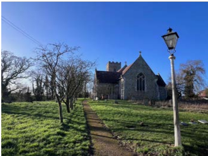
d View west through the churchyard from Church Lane to St Peter's Church.
