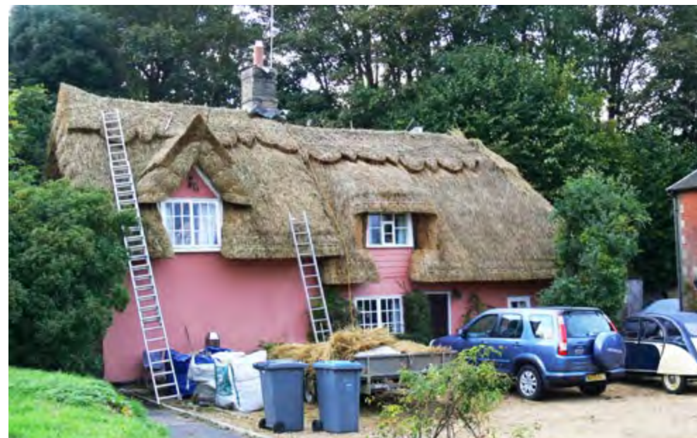
A new thatch, being applied to a timber framed, rendered and colour-washed cottage.
