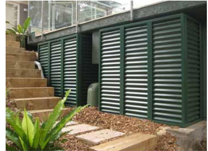
Figure 72: Concealed tanks integrated with the design.
